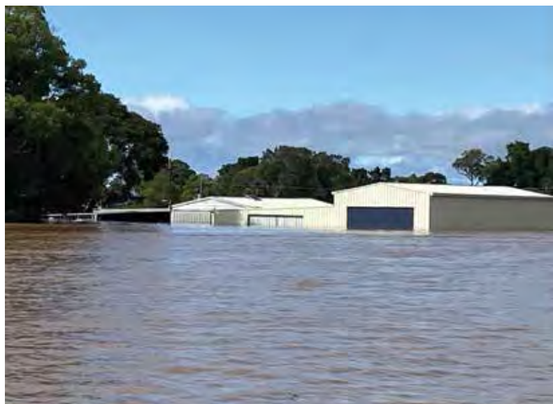
The main shed housing all the farm machinery was built higher than development requirements but still was flooded. In front of the shed are two-year-old trees under the water.
